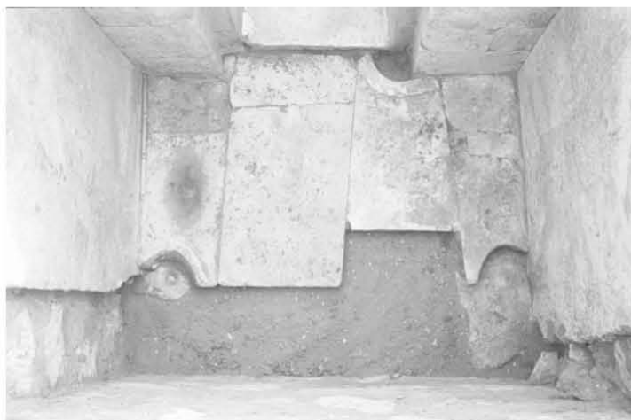
a) The chapel of Hetepi with postholes left behind by a two leaved door in front of the destroyed west wall.
