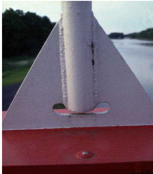
Figure 3.36: Hanger connection plate
