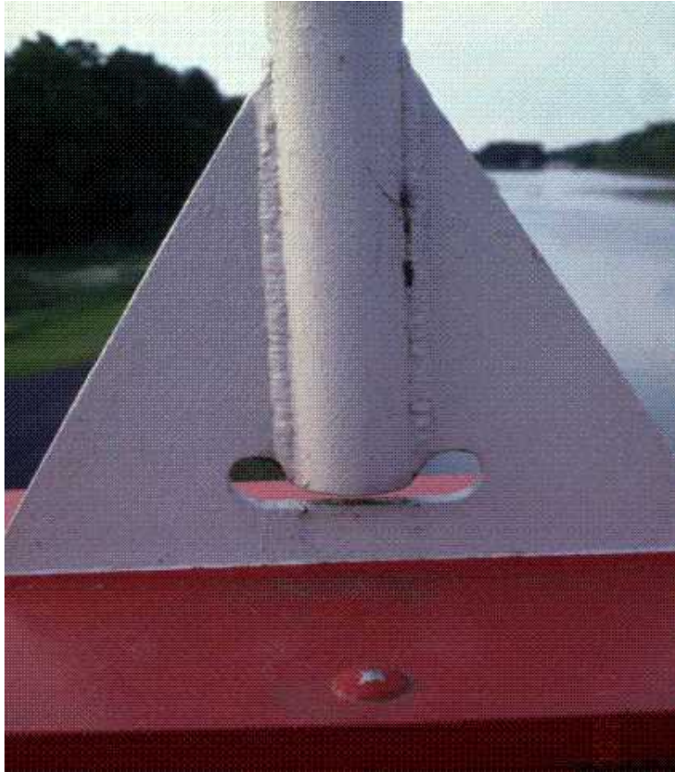
Abb. 4.21. Hanger connection plate
