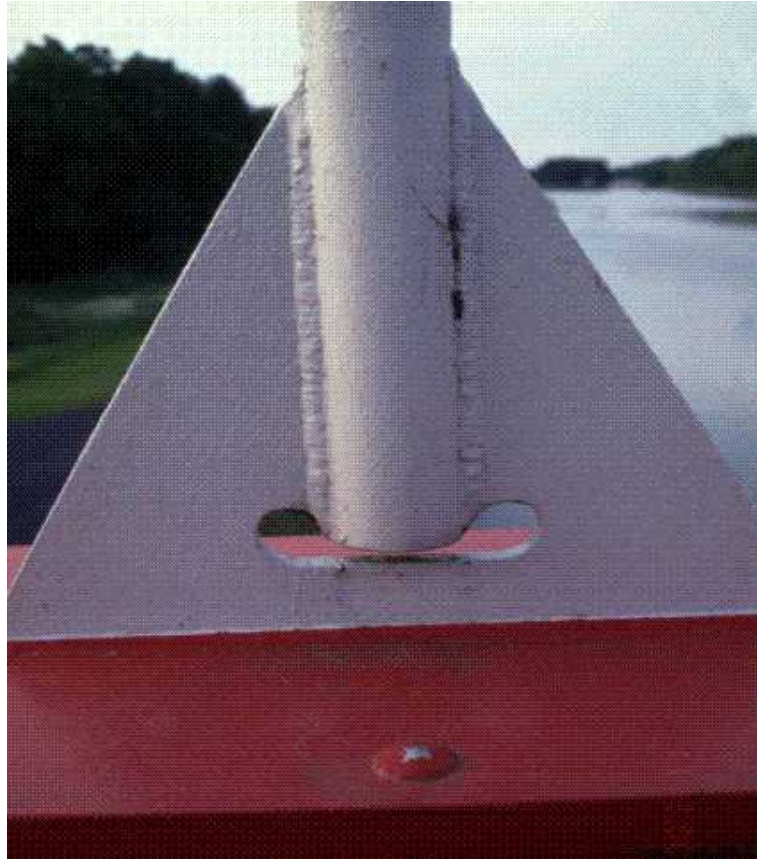
Figure 3.36: Hanger connection plate
