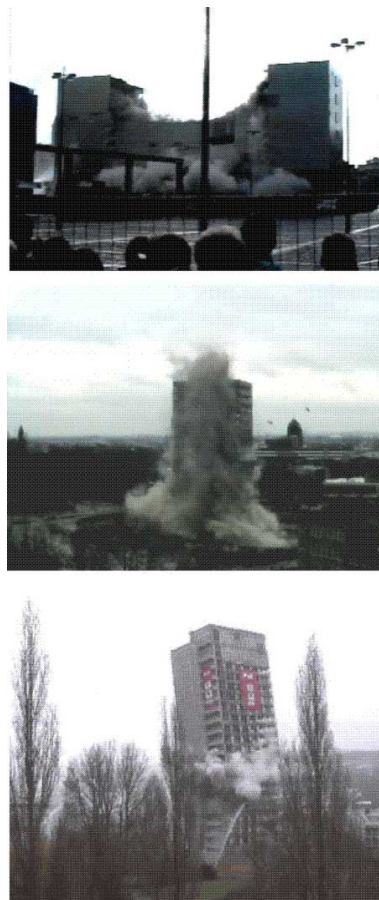
Figure 3.42: Instances of explosions in the practise
